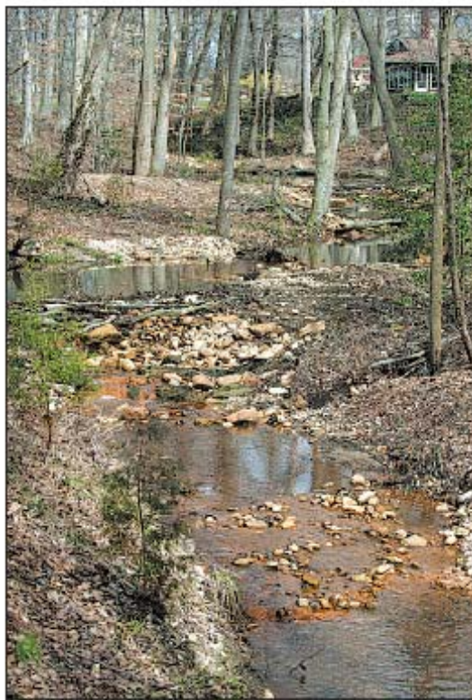
ABOVE: Dick Lahn of Crofton discusses the environmental impact of stormwater during a tour of the Beaver Creek watershed. LEFT: On the other side of Crofton Parkway, this section of Beaver Creek underwent over $600,000 in rehabilitation with a series of weirs and buffers designed to slow down water, increasing absorption into the ground.
