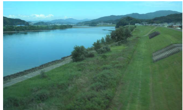
Protected levees along the Shimanto River
