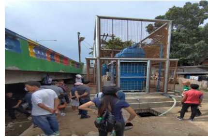
Figure 10. MSTP installed at Calubihan portion of Dungon Creek
