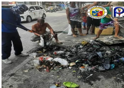
Figure 14. Declogging of city drainages
