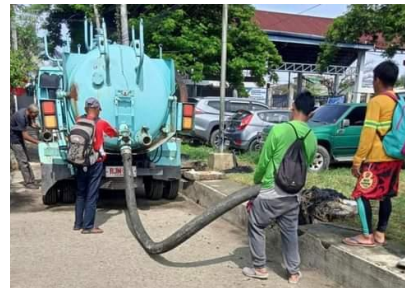
Figure 15. Vacuuming of city drainages
