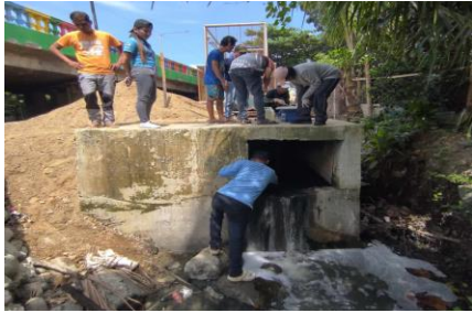
Figure 9. Interceptor installed at Calubihan portion of Dungon Creek
